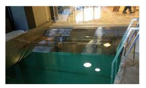
Stainless Steel Basin Bowl (DIN 316). In developing the basin bowl and spa area there were many unusual solutions used such as the system drain and water supply in the basin bowl: it's implemented through the slotted nozzles hidden from the pool users. There is also a pool ladder concealed in the walls and a combined triple hot zone where possibilities of combining pneumatic (middle zone) and hydraulic (marginal seats) massages with separate switches were created.
