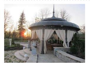
An arbor. The columns simulate highly accurate casting; unconventional brackets, thread sheathing beneath the roofing sheets prove the high quality of the product. The roof is constructed from volumetrically deformed copper sheets.
